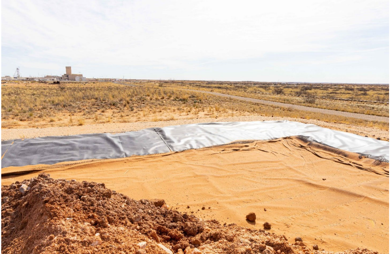
Figure 2 New Salt Storage Cell for SSCVS, Photography by Roy Neese
