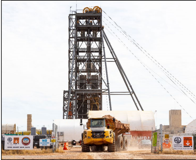
Figure 1 – Utility Shaft Number 5, Photography by Roy Neese
